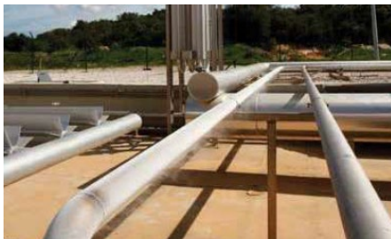
Construction gas network – Portugal 450K€
