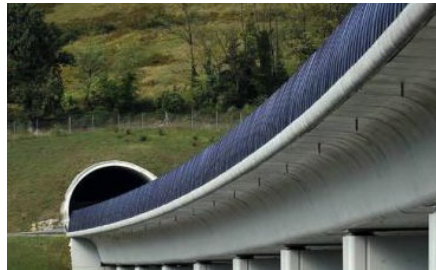
High-speed Pamplona-Zaragoza – Spain 17M€
