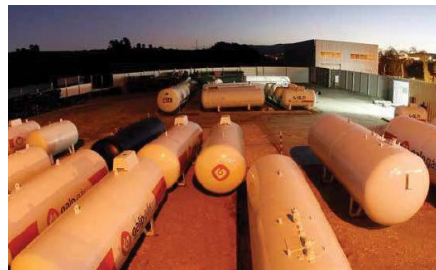
Refurbishment of lpg tanks – Portugal 800K€
